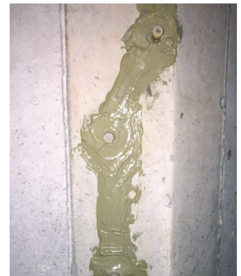
Conventional injected crack
